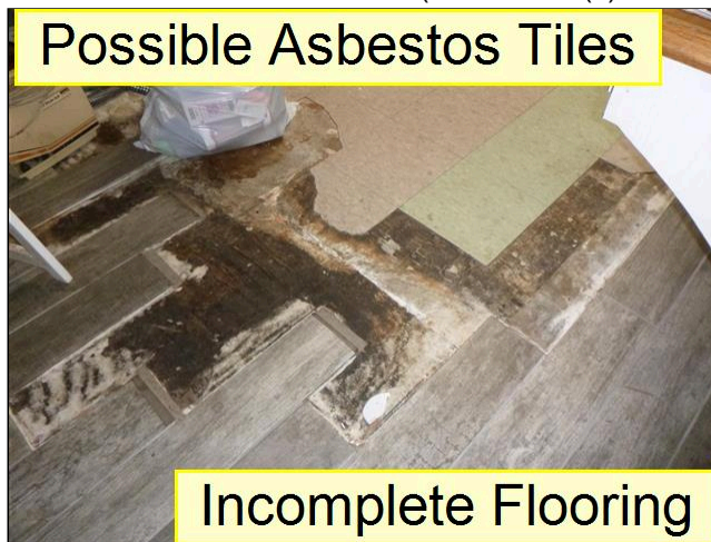
Stains/Water Damage
