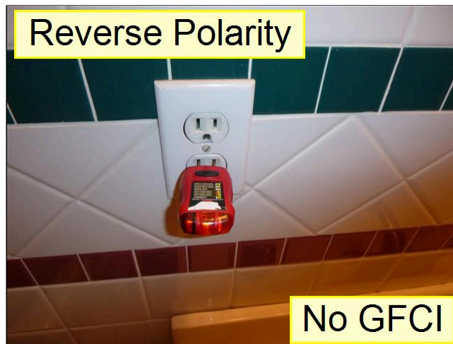
6.5 ELECTRIC / GFCI (See Picture(s))
