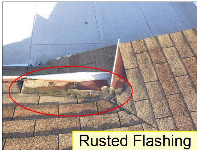
1.1 EXPOSED FLASHING (See Picture(s))
