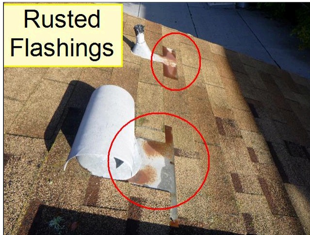
1.1 EXPOSED FLASHING (See Picture(s))
